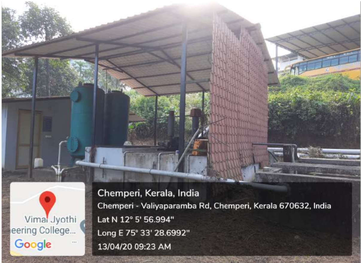
Figure: Aerobic Water treatment system- Pumping Unit area
