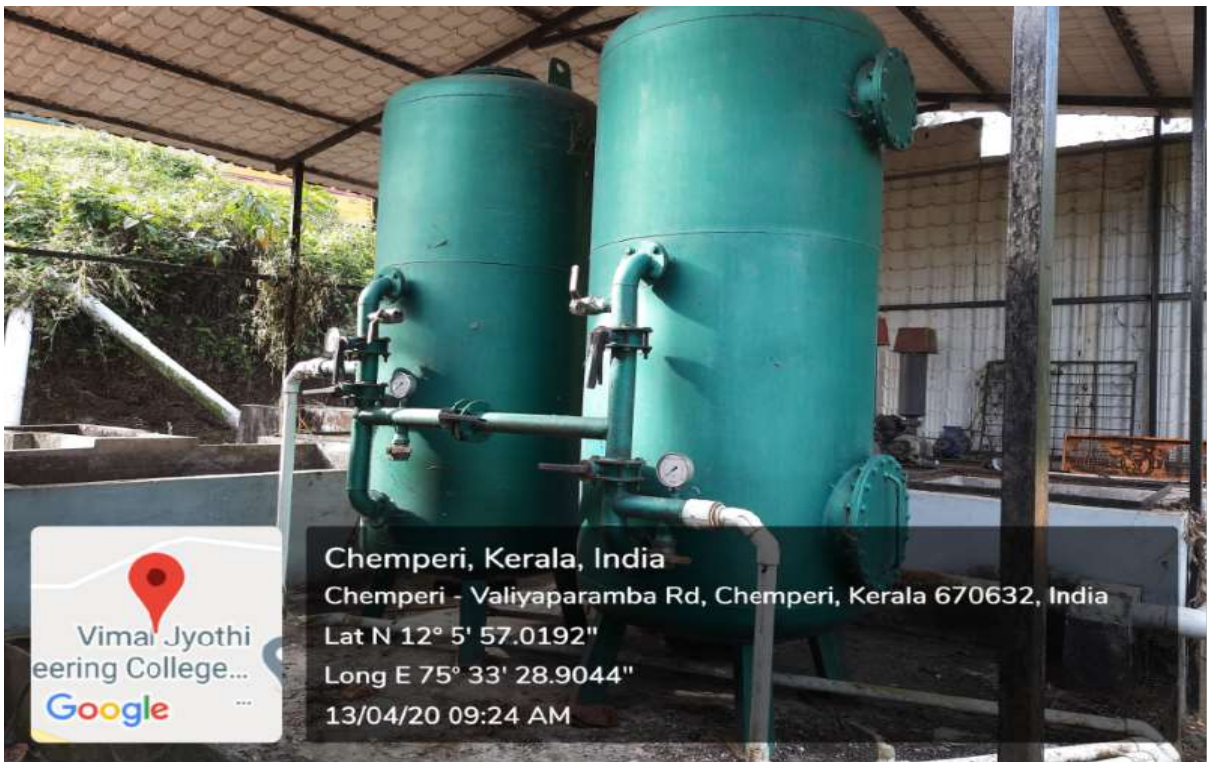
Figure: Aerobic Water treatment system- Aeration and filtering unit area
