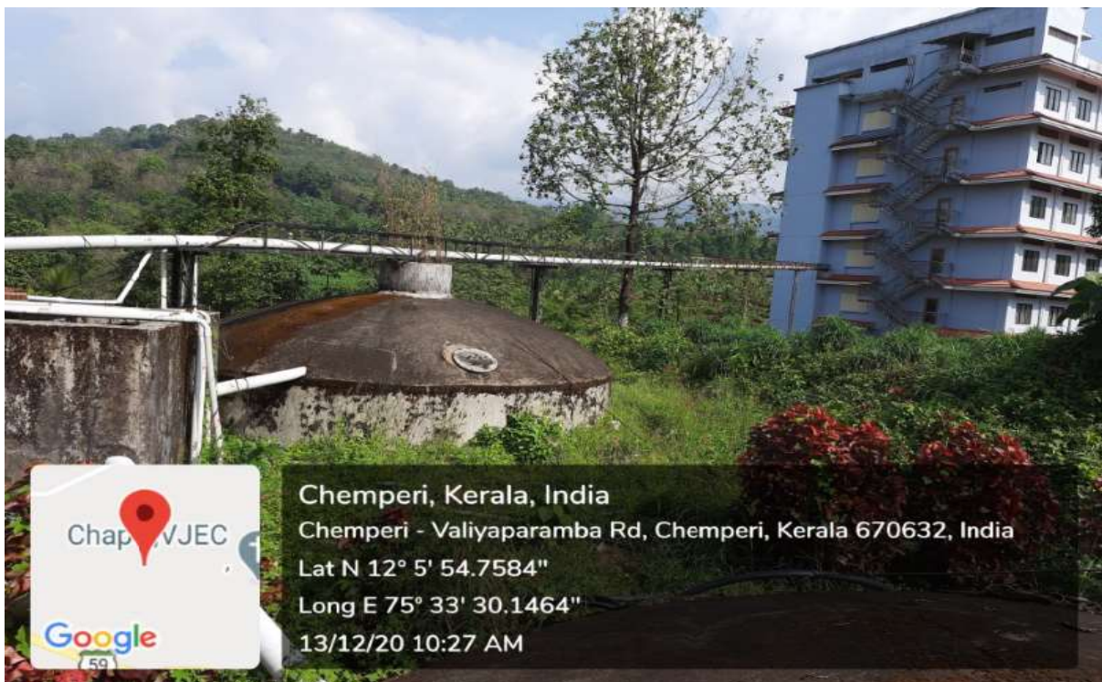
Figure: Integrated rain water tanks for rain water Harvesting.
